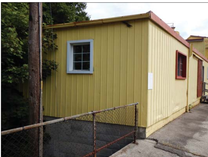
Photo 41 - September 20, 2022 Neustadt Dam and Flood Control Wall Building on Left Bank
