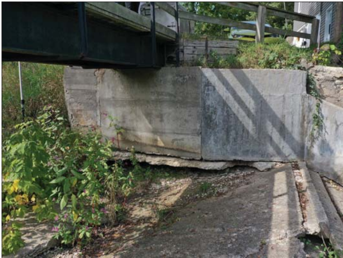
Photo 25 - September 20, 2022 Neustadt Dam and Flood Control Wall Right Side Retaining Wall
