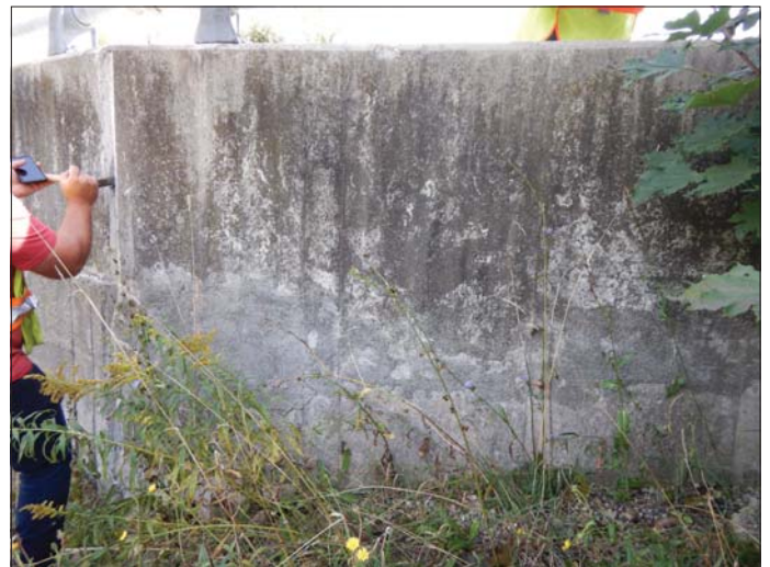
Photo 4 - September 20, 2022 Neustadt Dam and Flood Control Wall Upstream Side of Flood Control Wall
