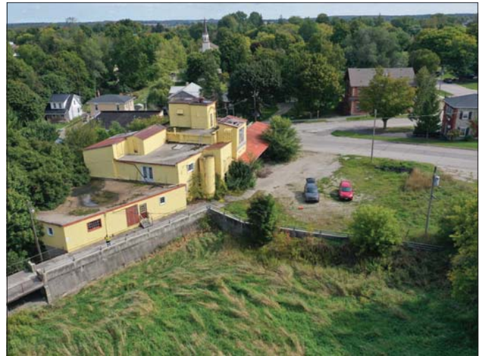
Photo 2 - September 20, 2022 Neustadt Dam and Flood Control Wall Aerial View of Flood Control Wall
