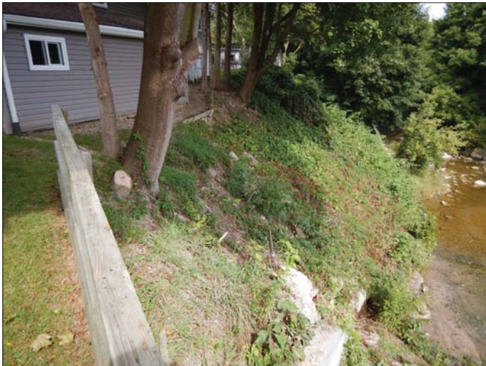
Photo 49 - September 20, 2022 Neustadt Dam and Flood Control Wall Downstream Right Bank
