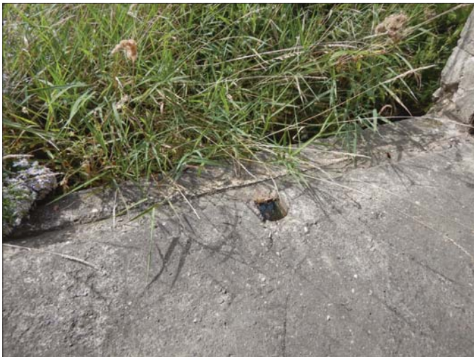
Photo 11 - September 20, 2022 Neustadt Dam and Flood Control Wall Control Structure, Sluice 1 Sill
