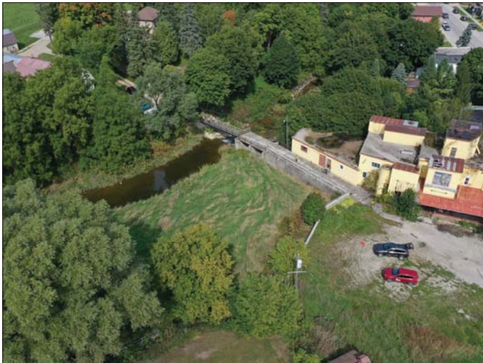
Photo 1 - September 20, 2022 Neustadt Dam and Flood Control Wall Aerial View of Upstream Side of Dam
