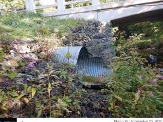
Photo 15 - September 20, 2022 Neustadt Flood Control Works - Meux Creek Culvert Outlet on Right Bank
