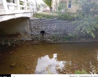
Photo 21 - September 20, 2022 Neustadt Flood Control Works - Meux Creek Gabion Baskets on Left Bank Upstream of Bridge
