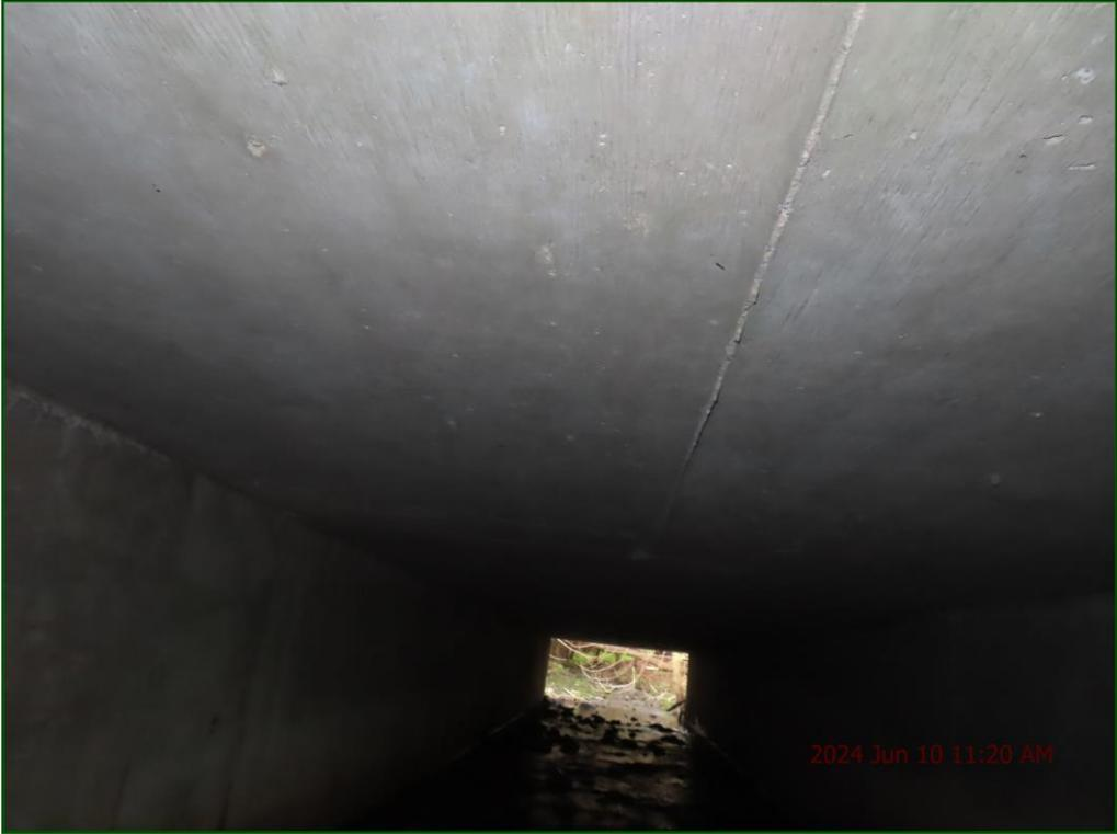
Description: Barrel: Shallow spalling with exposed reinforcing.
