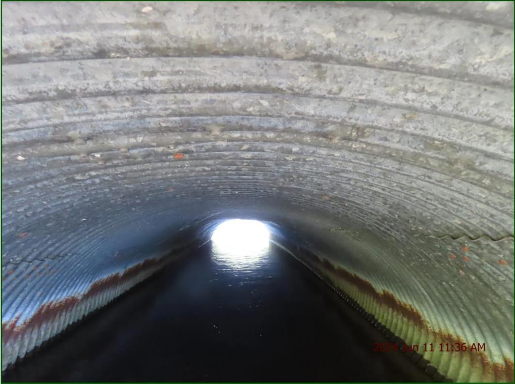
Description: Inlet: Severe scouring of south barrel.
