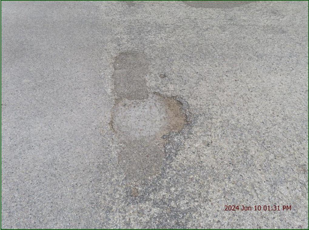
Description: Wearing surface: Severe alligator cracking at shoulders.
