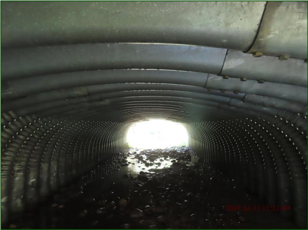
Description: Barrel: Minor deformations in barrel.
