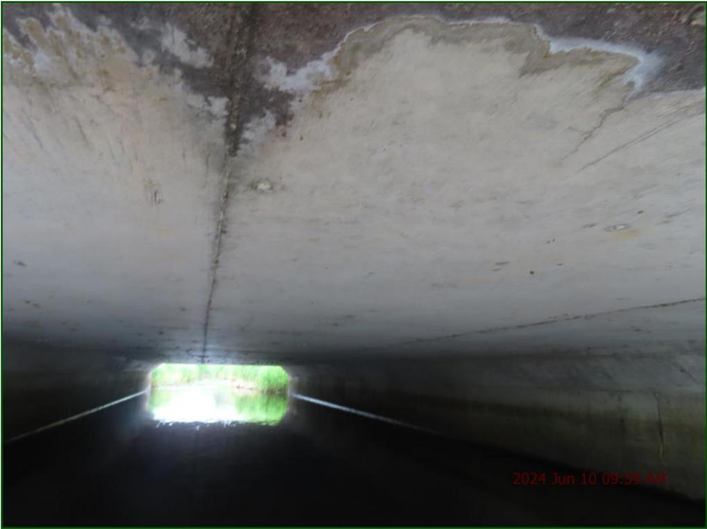
Description: Barrel: Medium longitudinal crack with leachate staining and stalactite (1/2).
