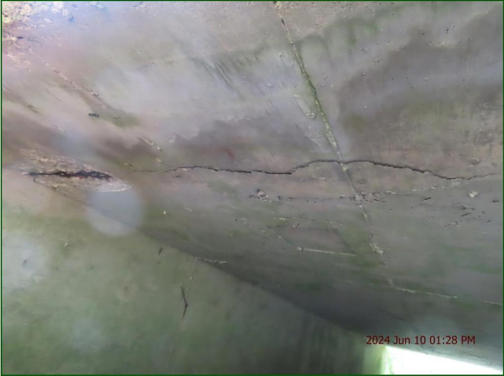
Description: Barrel: Shallow localized spall with exposed reinforcing.
