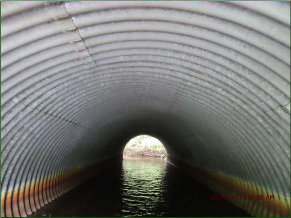
Description: Barrel: Improper splice bolt pattern, no cracking noted.
