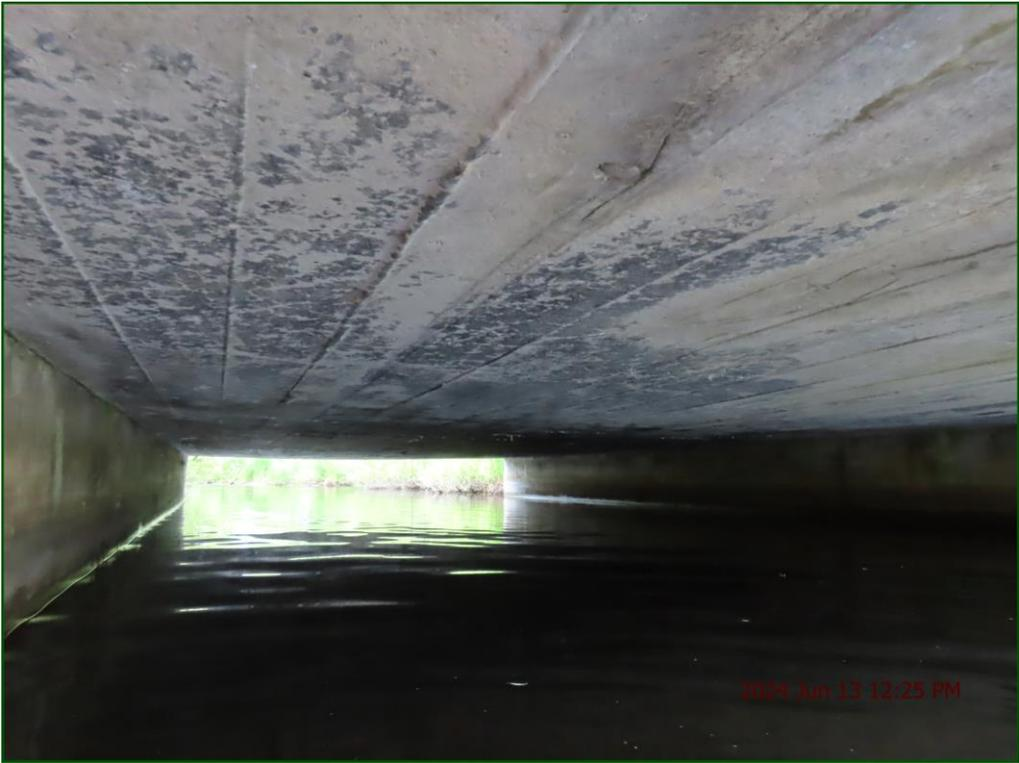
Description: Inlet: Medium cracking at construction joints, possible sign of inward rotation.
