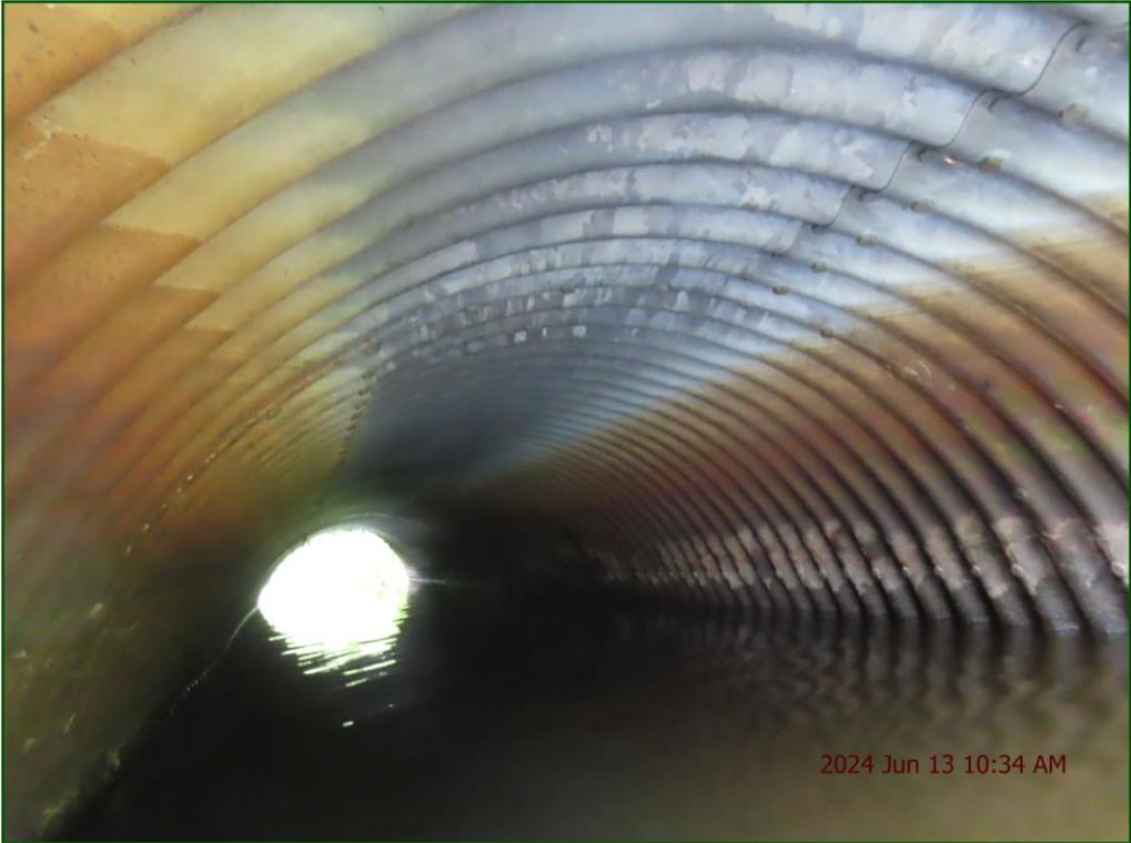
Description: Wearing surface: Moderate erosion at edges.
