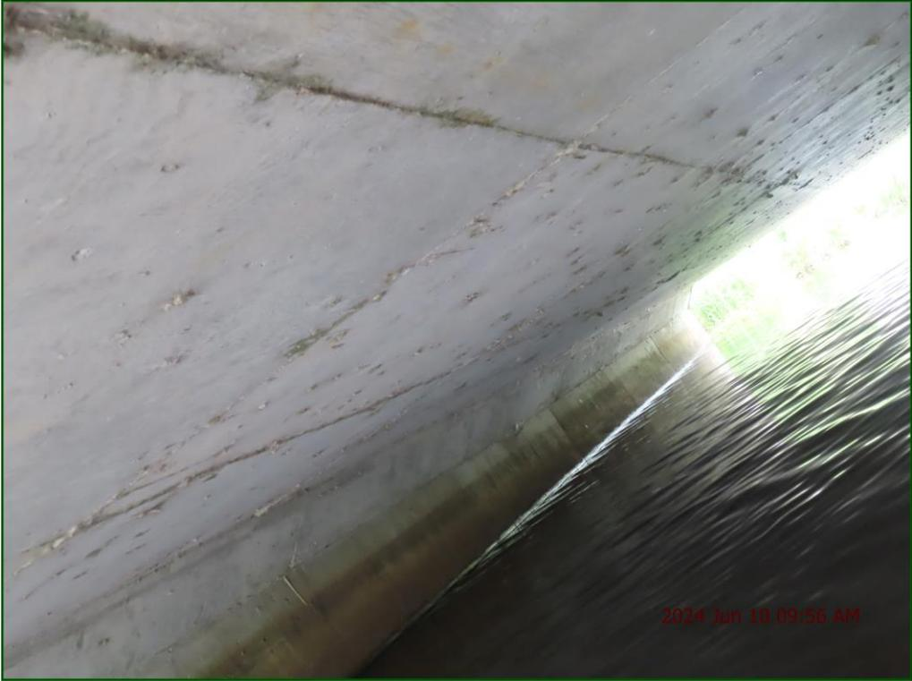
Description: Inlet: Medium horizontal crack.
