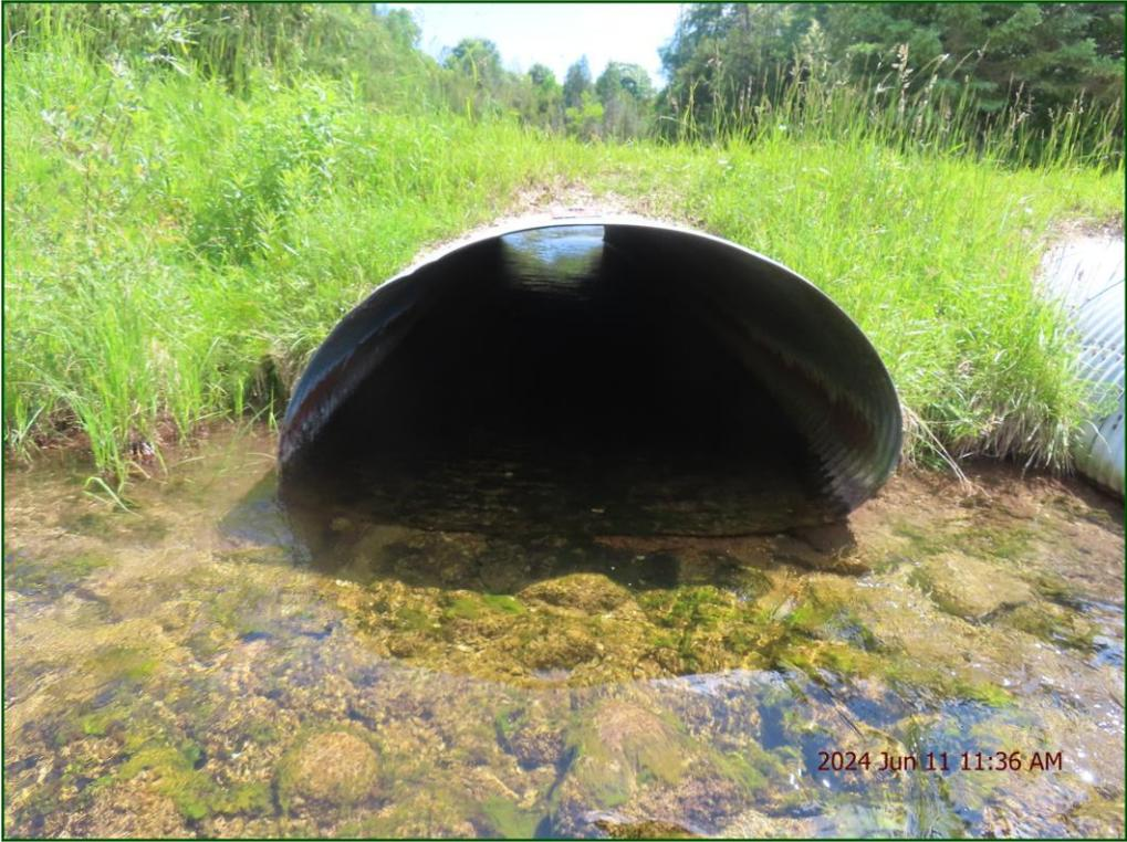
Description: Barrel: Moderate deformation mid barrel.
