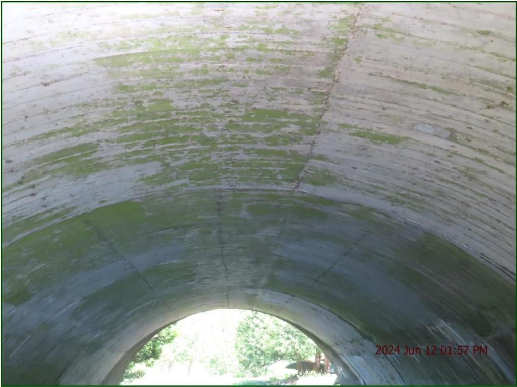
Description: Barrel: Medium to wide transverse cracks with leachate staining (1/2).
