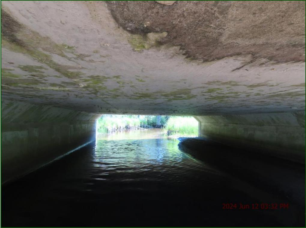
Description: Inlet: Light to medium cracking with leachate staining.
