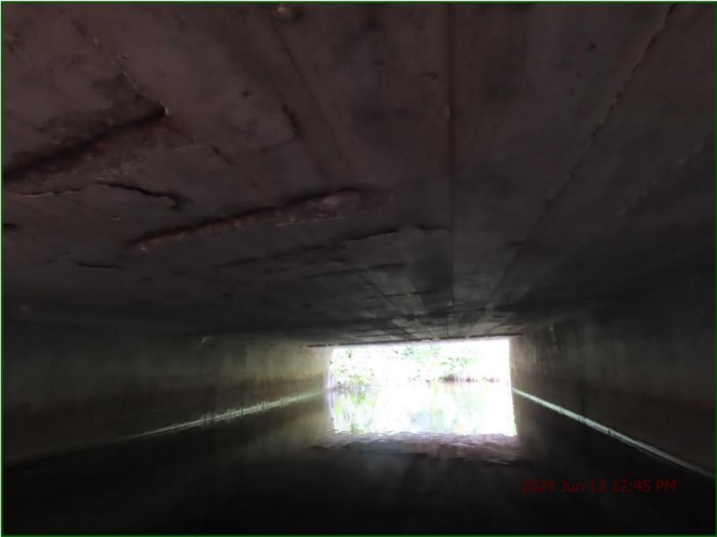
Description: Barrel: Shallow to severe delaminations with exposed reinforcing throughout.
