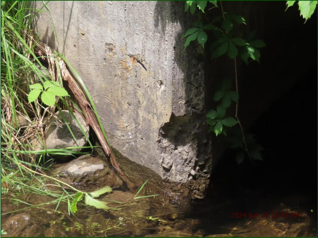
Description: Inlet: Light horizontal cracking with leachate staining.
