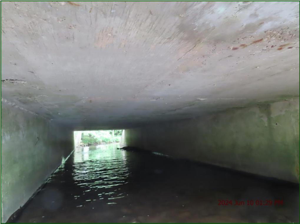
Description: Barrel: Light vertical cracks with wetness and leachate staining.
