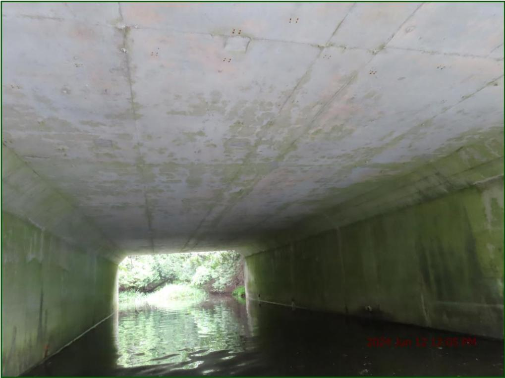
Description: Barrel: Light to medium vertical cracks with leachate staining.
