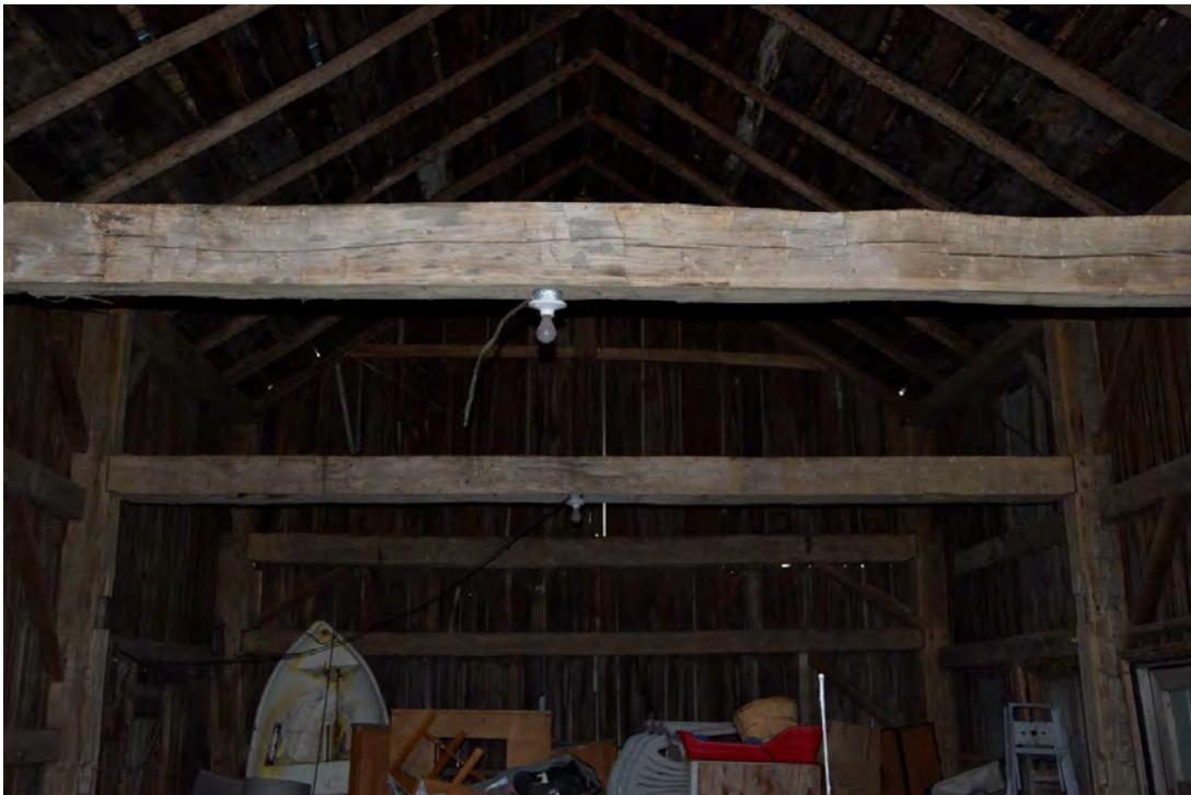
FIGURE 28: INTERIOR CONSTRUCTION OF SMALLER TIMBER FRAME STRUCTURE
