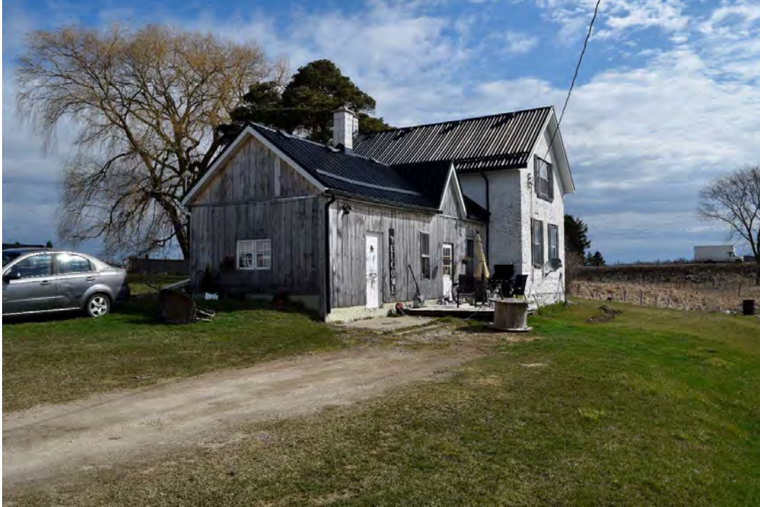
FIGURE 13: SOUTHWEST CORNER WITH FOCUS OF REAR ADDITION, FACING EAST-NORTHEAST
