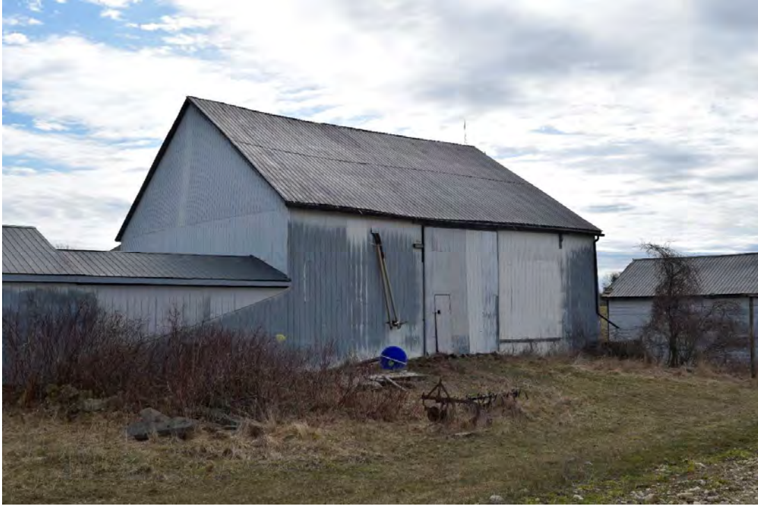
FIGURE 23: WEST FACE OF BANK BARN, WITH ACCESS RAMP
