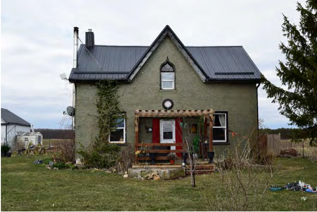
FIGURE 34: FRONT FAÇADE, FACING WEST
