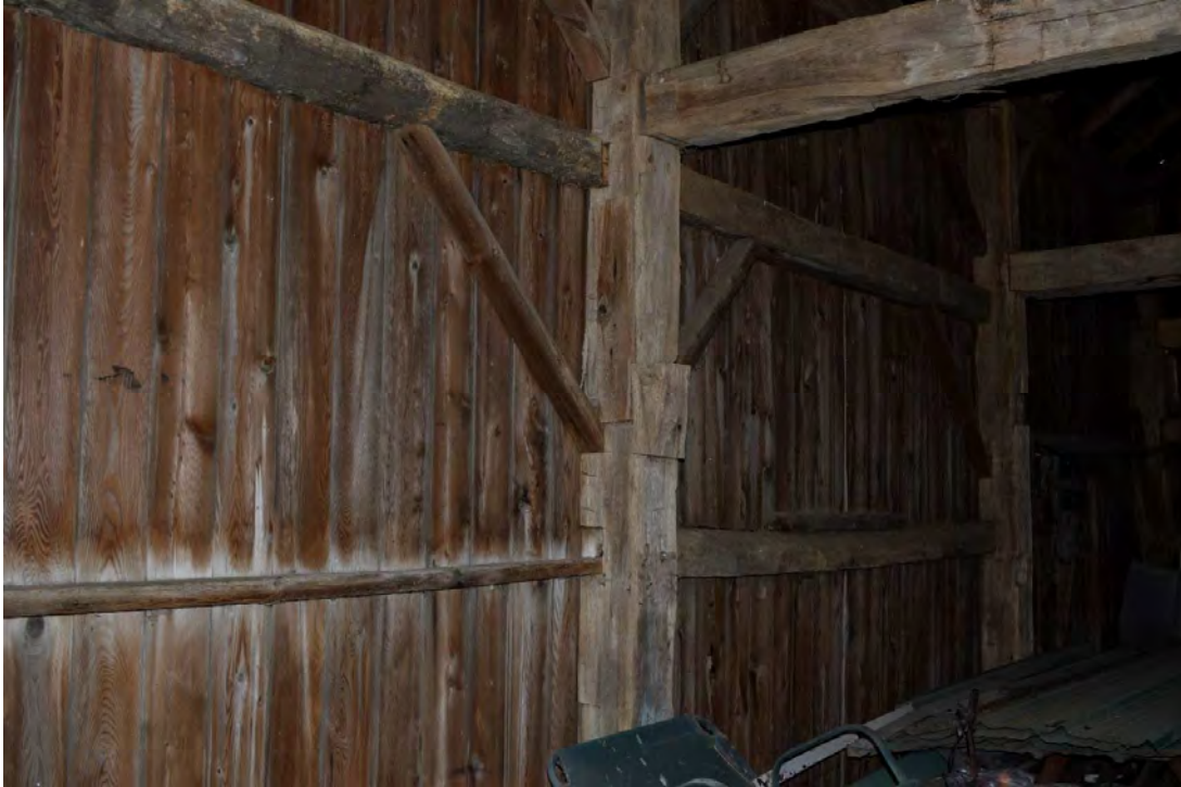
FIGURE 29: CLOSEUP OF INTERIOR OF SMALLER TIMBER FRAME STRUCTURE
