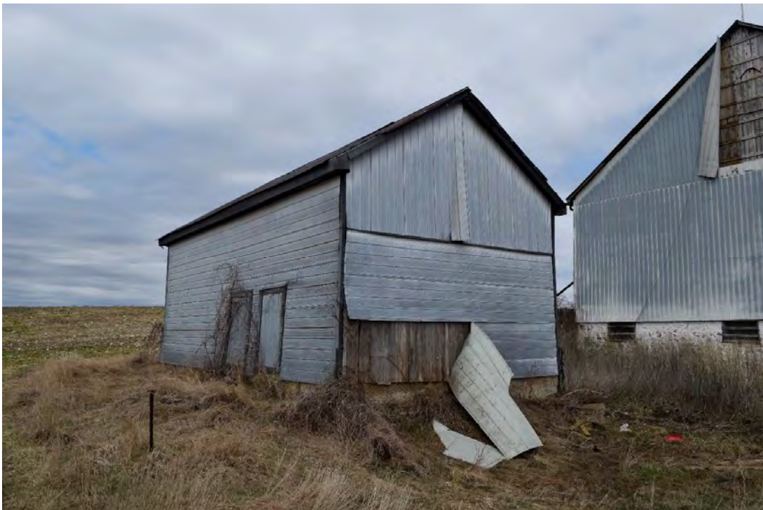
FIGURE 26: SMALL FREESTANDING TIMBER FRAME STRUCTURE
