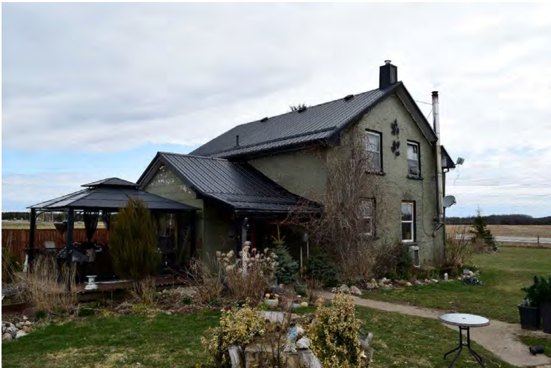
FIGURE 37: SOUTHWEST EXPOSURE, FACING NORTHEAST
