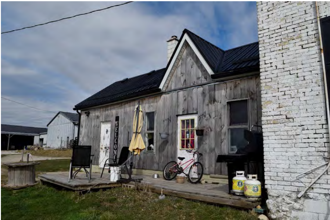
FIGURE 14: SOUTH FACE OF REAR ADDITION, FACING NORTHWEST
