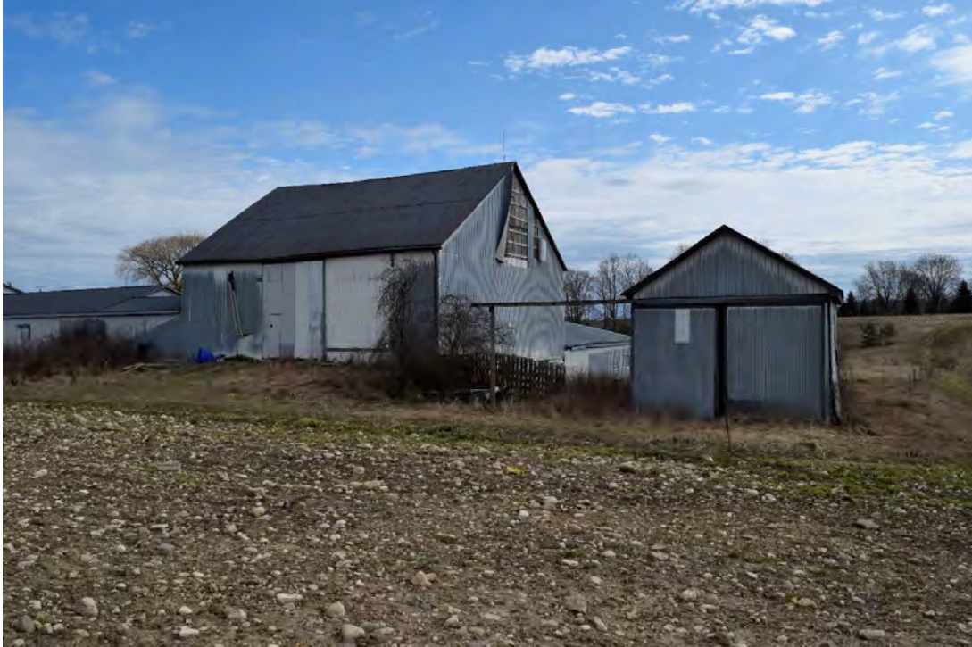
FIGURE 25: BANK BARN IN RELATION TO SMALLER FREESTANDING TIMBER FRAME STRUCTURE
