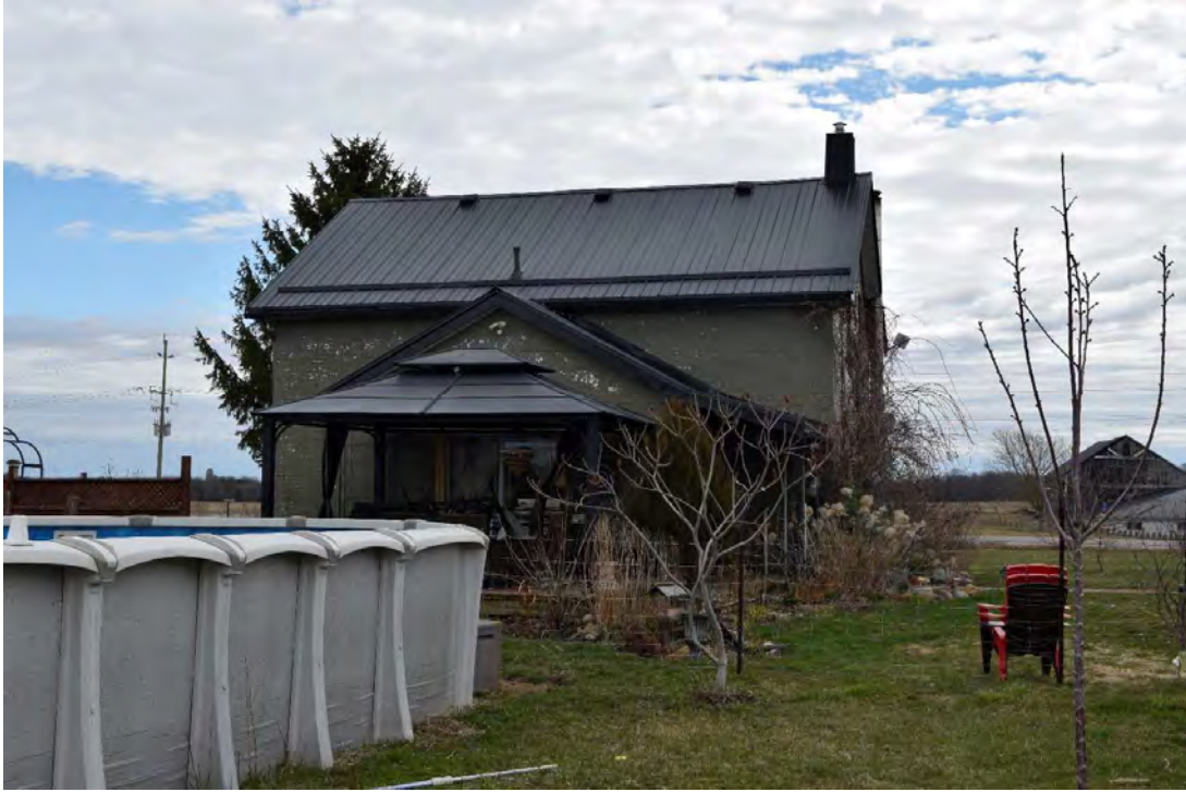
FIGURE 38: WEST EXPOSURE WITH REAR ADDITION, FACING EAST
