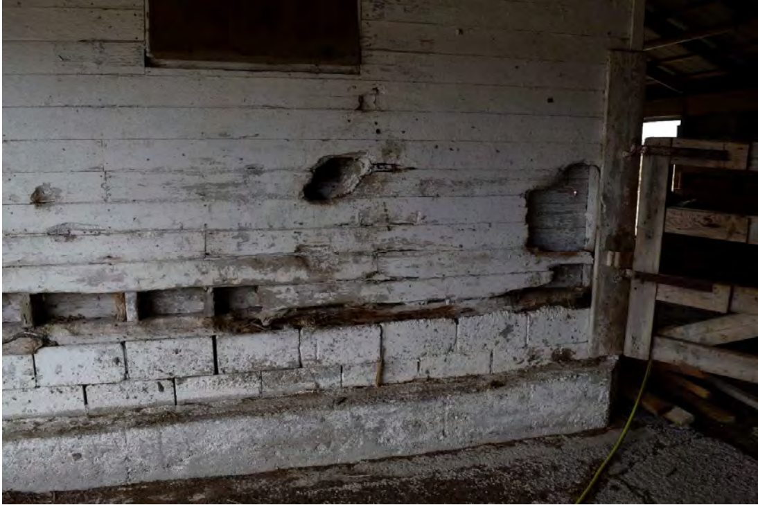
FIGURE 49: CONCRETE AND CONCRETE BLOCK FOUNDATION OF MID-20 TH CENTURY OUTBUILDING
