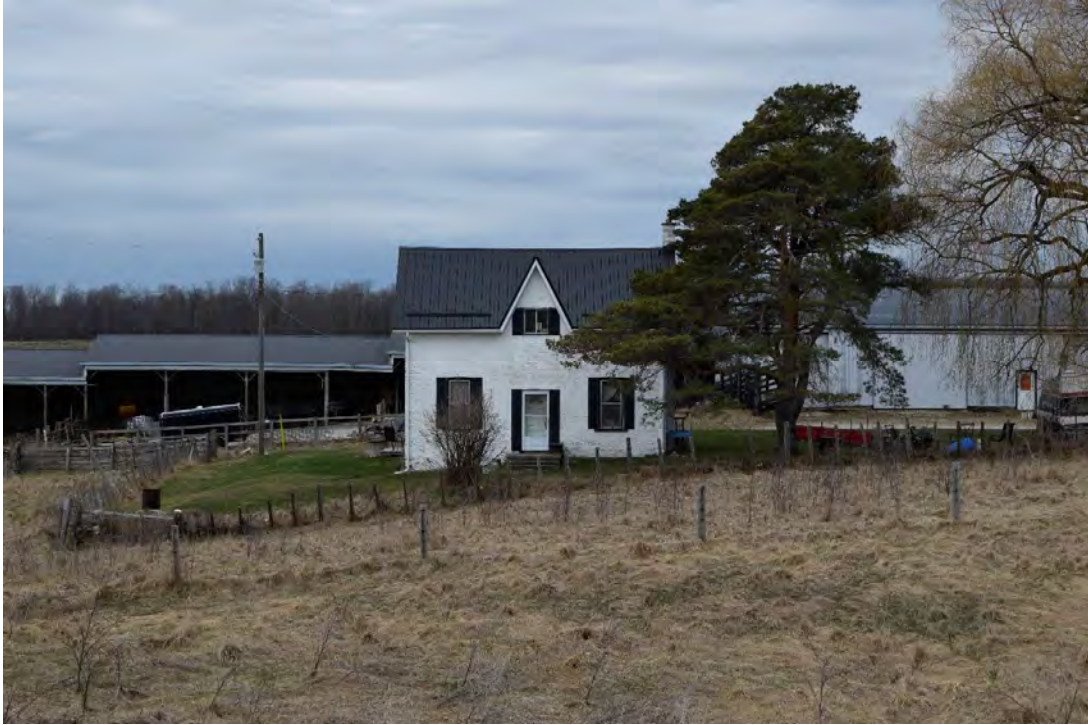
FIGURE 7: FRONT FAÇADE AS SEEN FROM HIGHWAY 6, FACING WEST
