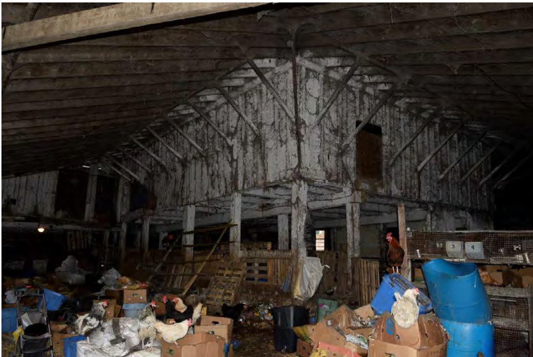
FIGURE 32: INTERIOR VIEW OF BANK BARN COMPLEX
