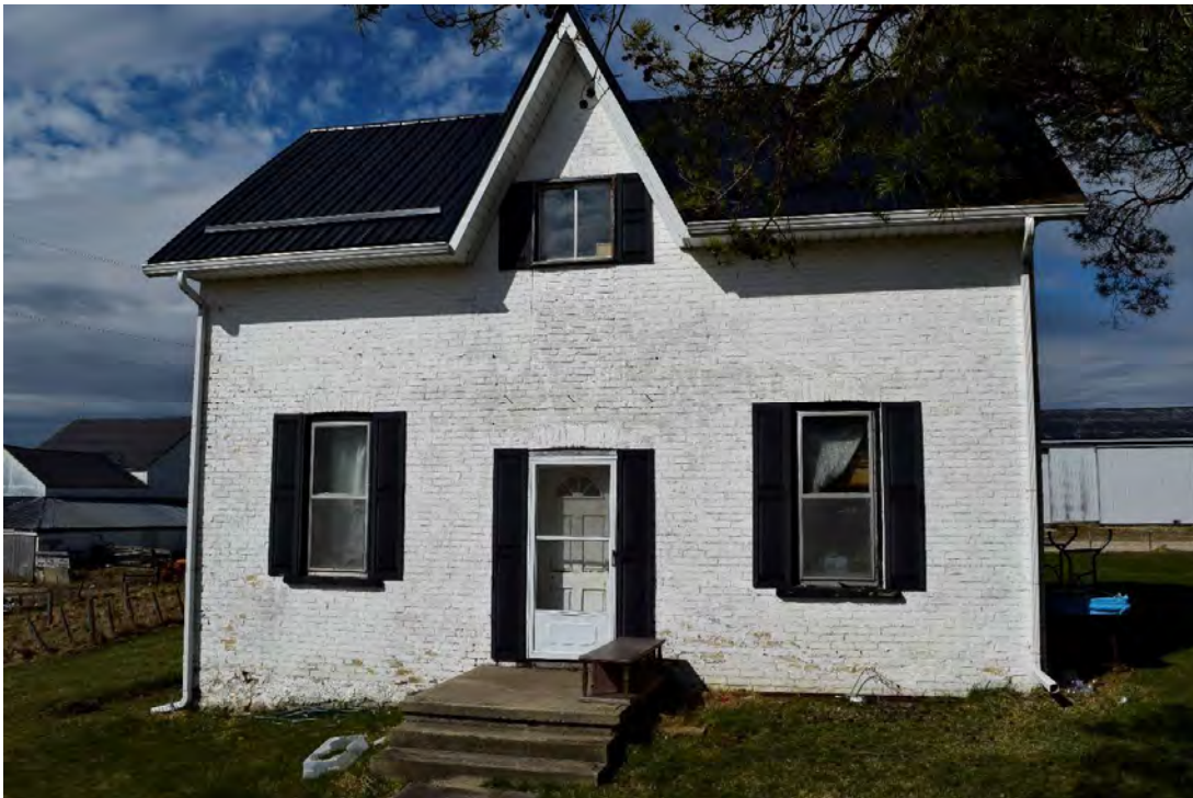
FIGURE 10: CLOSE UP OF FRONT FAÇADE, FACING WEST
