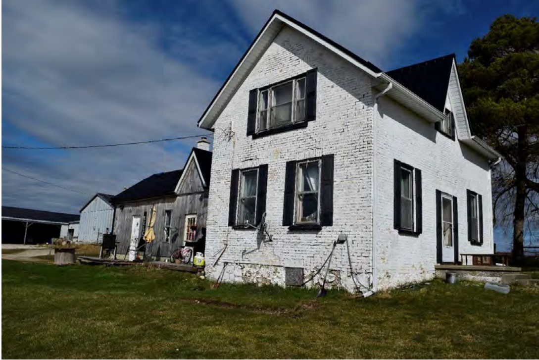
FIGURE 9: SOUTHEAST CORNER, FACING NORTHWEST
