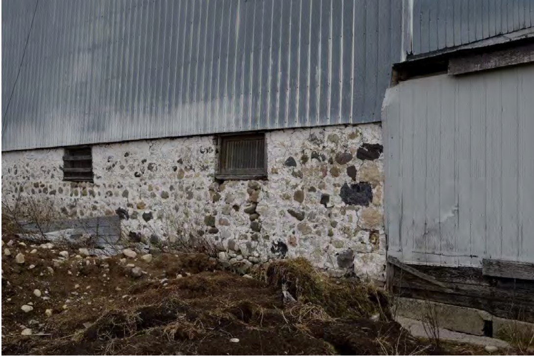
FIGURE 31: FIELD STONE FOUNDATION OF BANK BARN
