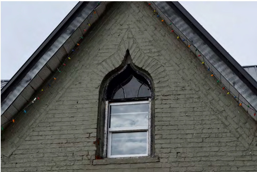
FIGURE 41: UNIQUE CIMA REVERSA OGEE WINDOW IN CENTER GABLE, NOTE DECORATIVE BRICK WORK AROUND WINDOW AND AT SOFIT
