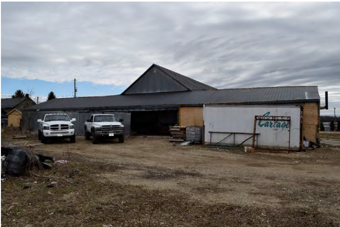
FIGURE 48: MID-20 TH CENTURY OUTBUILDING, WEST FACE DEPICTING LATER ADDITION
