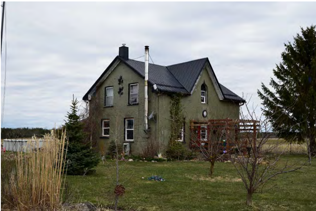
FIGURE 35: SOUTHEAST EXPOSURE, FACING NORTHWEST
