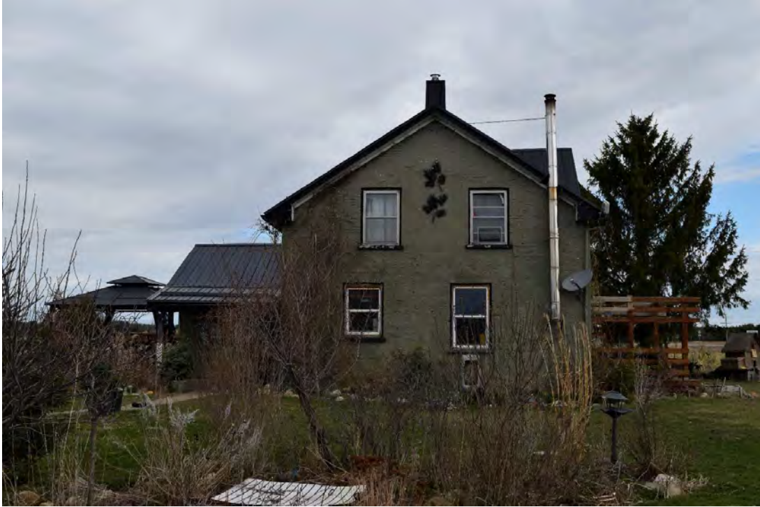
FIGURE 36: SOUTH FACE, FACING NORTH
