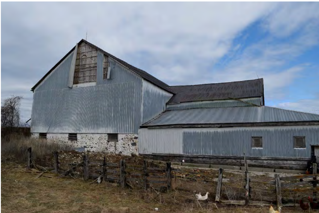
FIGURE 24: NORTH FACE OF BANK BARN
