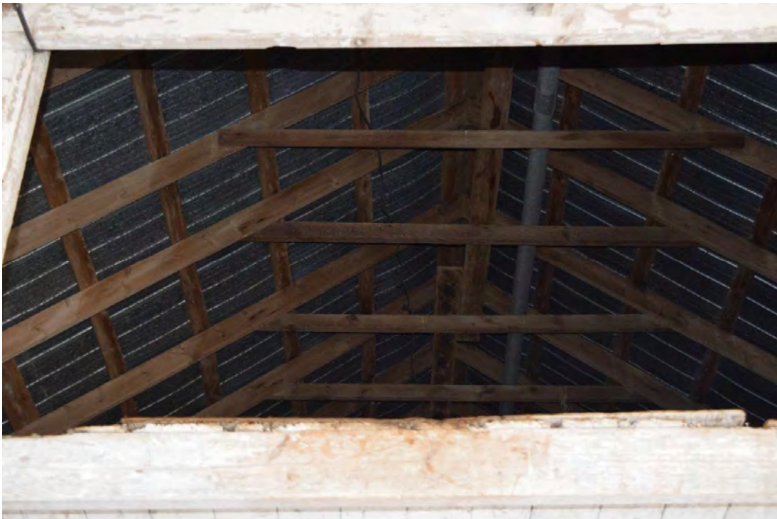
FIGURE 50: ROOF STRUCTURE OF MID-20 TH CENTURY OUTBUILDING
