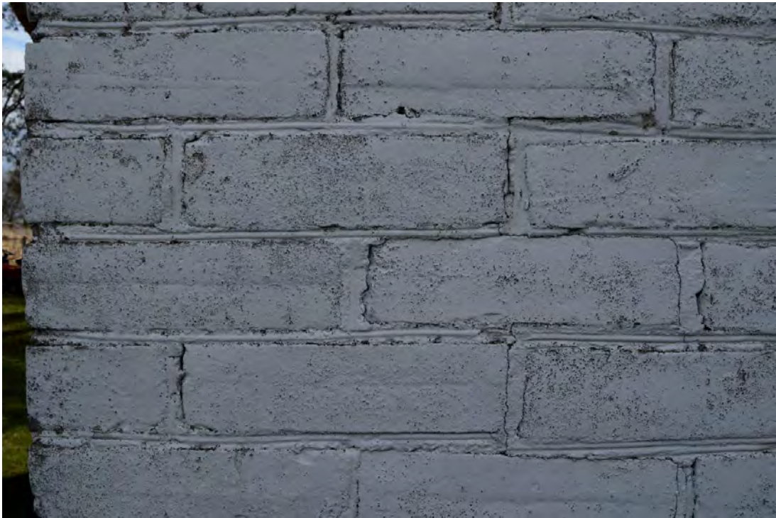
FIGURE 18: EXAMPLE OF ORIGINAL TOOLED MORTAR JOINTS BETWEEN BRICKS
