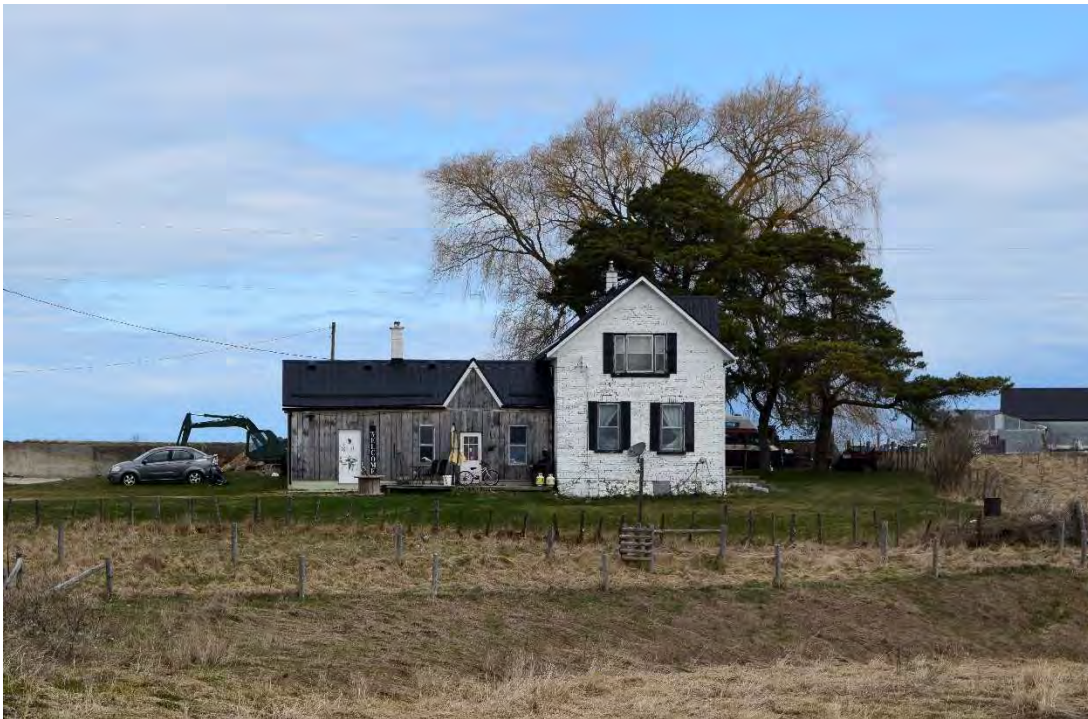
FIGURE 8: SOUTH FACE, FACING NORTH
