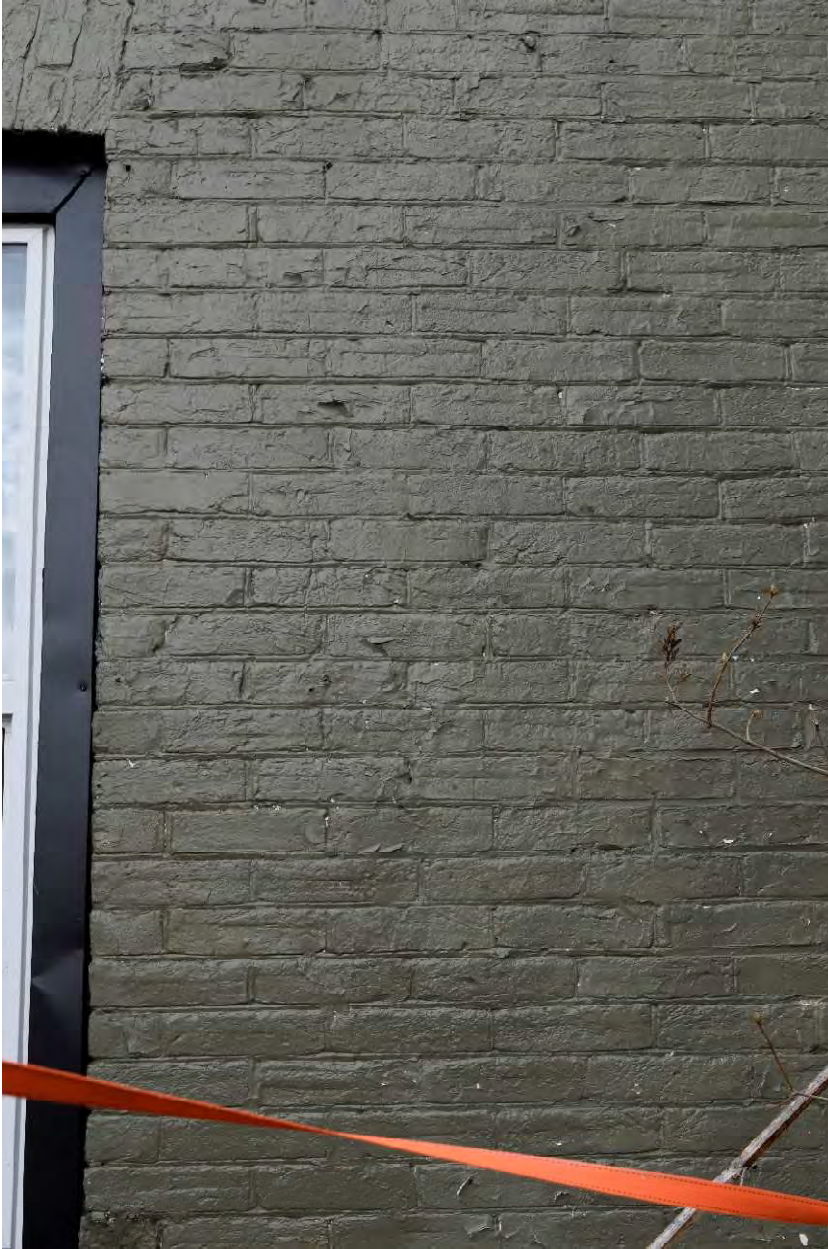
FIGURE 42: TYPICAL EXAMPLE OF TOOLED MORTAR JOINTS BETWEEN BRICKS
