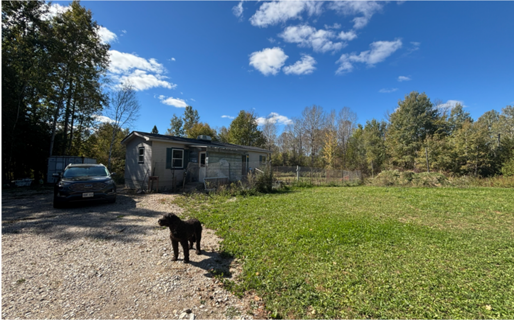
Photo 1 - South West-facing view of onsite building.
