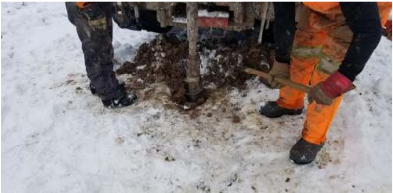
Photo 2 - Drilling of MW-4 (February 23, 2021)
