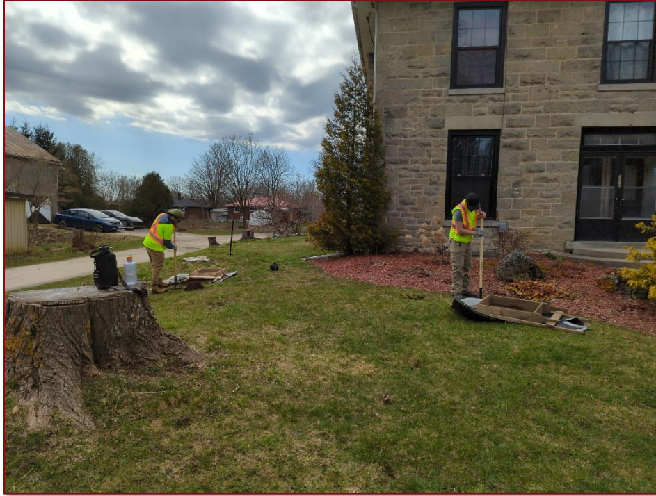
Image 4: Typical Test Pit
