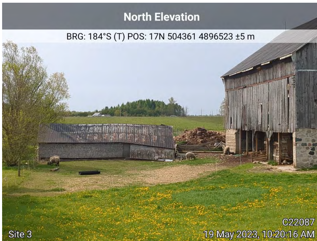
Photo 1: Operation #3 – Hobby farm showing sheep, barn, and outdoor manure storage
