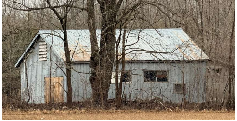
Eastern façade from Bell's Lake Road
