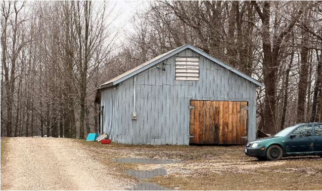
Front view of Structure from Bell's Lake Road
