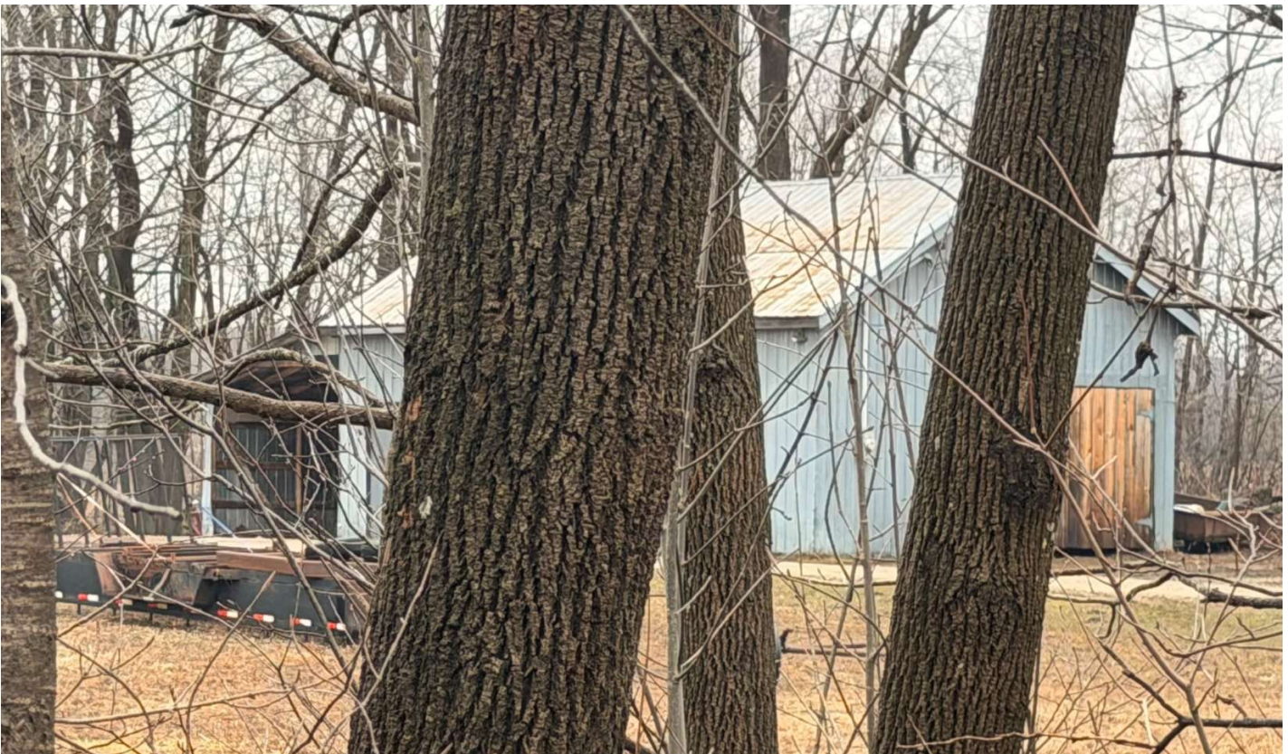
View of West façade and open lean to from Bell's Lake Road
